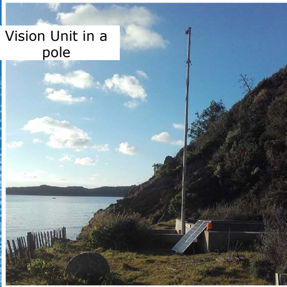
Computer Unit and Solar Panels installation
